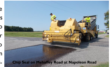
Chip Seal on Mehaffey Road at Napoleon Road
