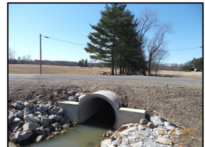
Pevee Road Bridge south of Hog Creek
