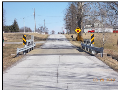
Faulkner Road Bridge west of Napoleon Rd
