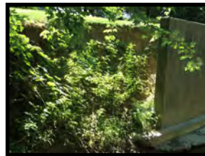
FLAT FORK DITCH EROSION PRE-GABION
