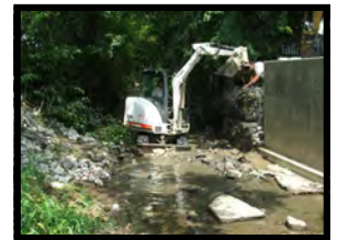
FLAT FORK DITCH GABION BASKET INSTALLATION
