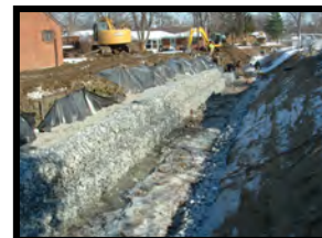
PIKE RUN DITCH GABION INSTALLATION
