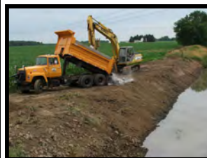
ROCK CHANNEL PROTECTION INSTALLATION
