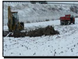
Agricultural Conduit Repair
