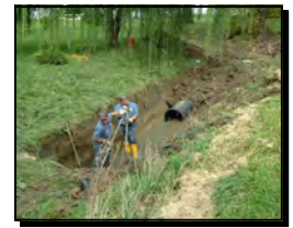
Residential Conduit Repair
