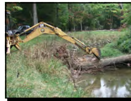
Log Jam & Debris Removal
