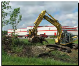
Flow line dip out & debris removal
