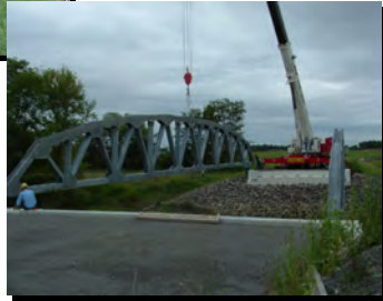
TOM FETT ROAD BRIDGE PLACEMENT OF TRUSS
