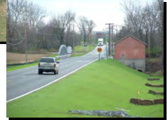
ROUSH ROAD BRIDGE (BEFORE)
